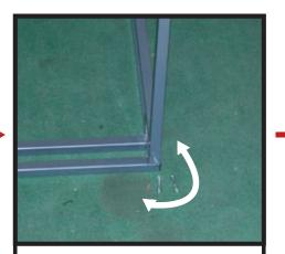
Line up pre-drilled holes and secure with bolt for parts 5 and 7 following the image above.
