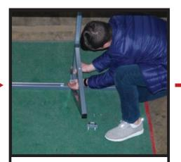
Line up part 17 with 16 and secure using two C-bracket, following the image above. Repeat for the remaining 17 parts.
