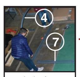
Once the piece from step 1 is facing up, place parts 4 and 7 (Left side) following the image above.
